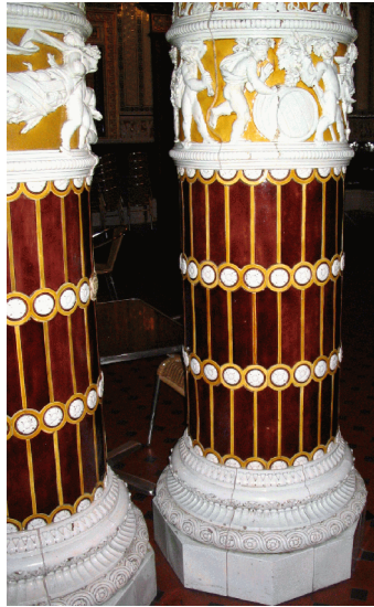
Figure 3-3: Centre Refreshment Room: majolica columns (lower drums).
