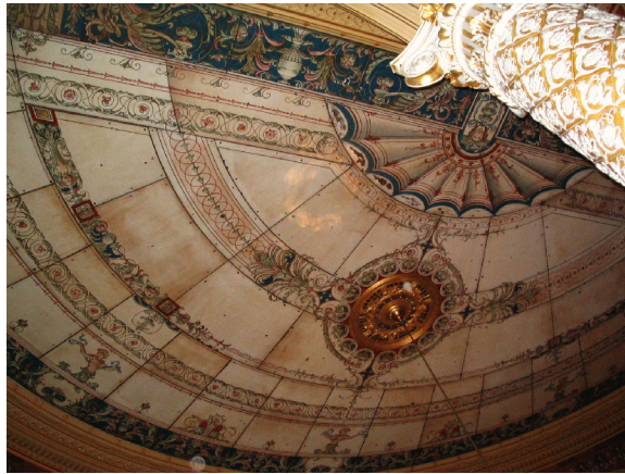
Figure 3-13: Centre Refreshment Room: a portion of the enameled iron ceiling.
